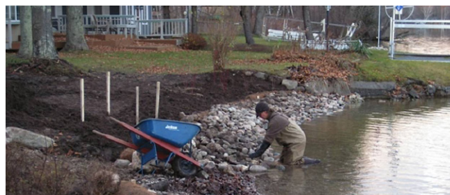
Biotechnical erosion control project being installed at a higher energy inland lake shoreline. Photos courtesy of Jennifer Buchanan, Tip of the Mitt Watershed Council.
